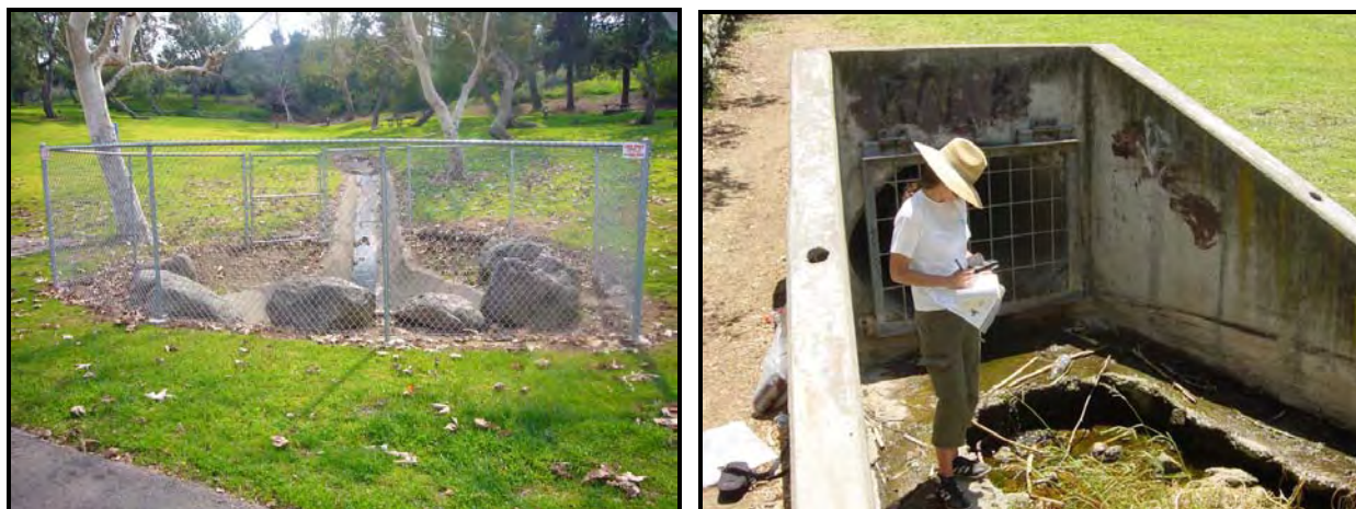
Figure 10-6. Storm Drain Discharges to Puddingstone Reservoir
